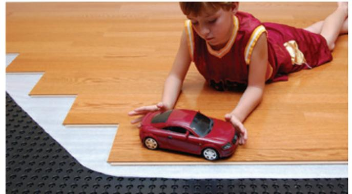
Virtually all basements have moisture problems. That's because moisture is continually released into homes through the concrete beneath the floor covering. Platon creates a moisture proof barrier and air gap between the floor and concrete, protecting the floor covering while allowing the concrete to breathe and the moisture to vent. As a result, the finished floor stays dry and warm, without build-up of mould, mildew or odours that affect the floor covering's lifespan and indoor air quality.
