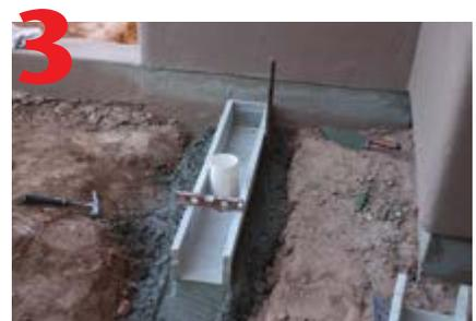
3 Lay channels starting at outlet. Set a string line at required height to ensure level.
