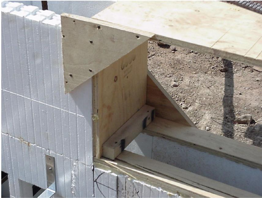
Figure 36 – Installing cleats around wall openings
