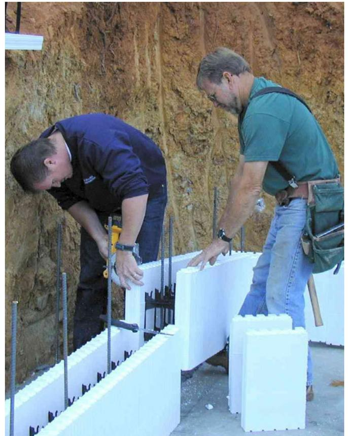
Figure 11 – Fitting the cut block in place
