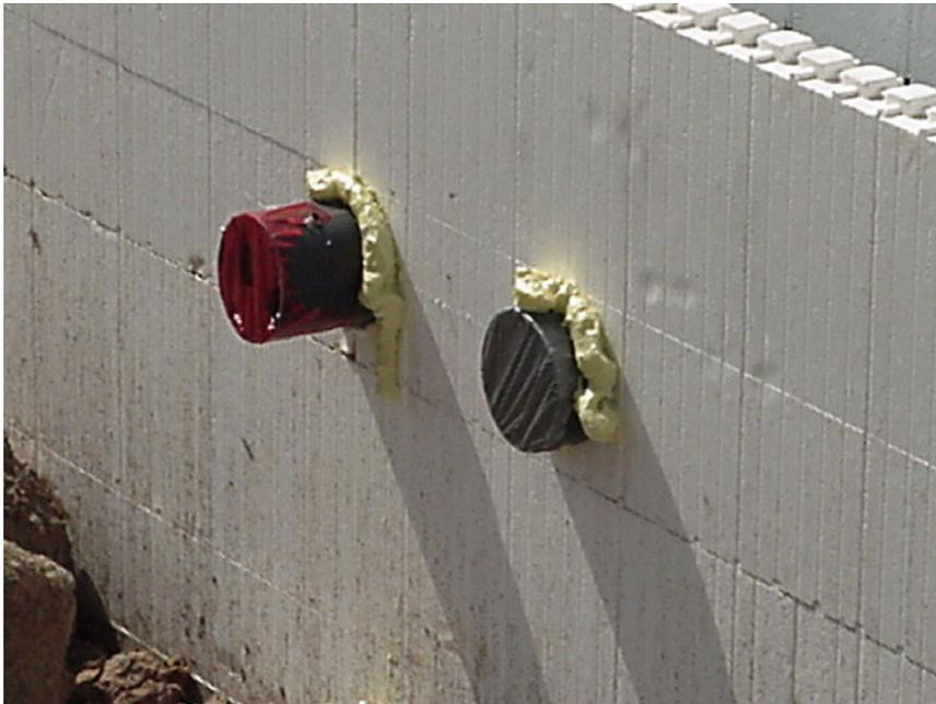
Figure 41 – Using PVC pipe for penetration block-outs
