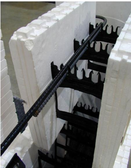
Figure 3 – Install horizontal reinforcing steel and lap splicing
