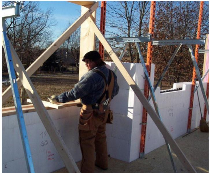
Figure 7 – Install alignment and bracing system around the interior of the perimeter wall
