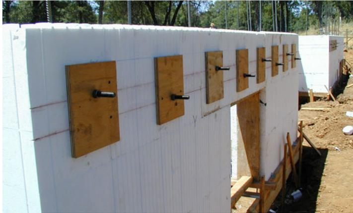
Figure 45 – Installing the OSB with anchor bolts onto the EPS openings and securing with drywall screws
