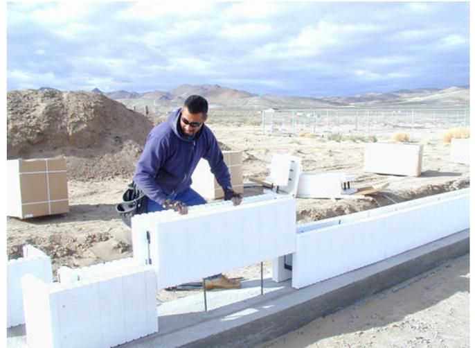
Figure 9 – Placing straight blocks
