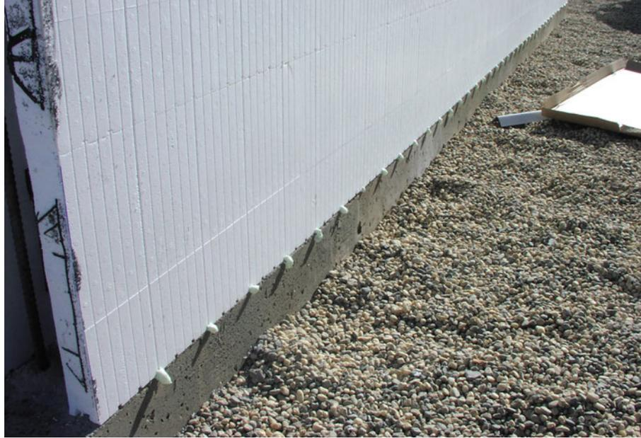
Figure 20 – Using foam adhesive to secure the first course of block to the foundation/slab
