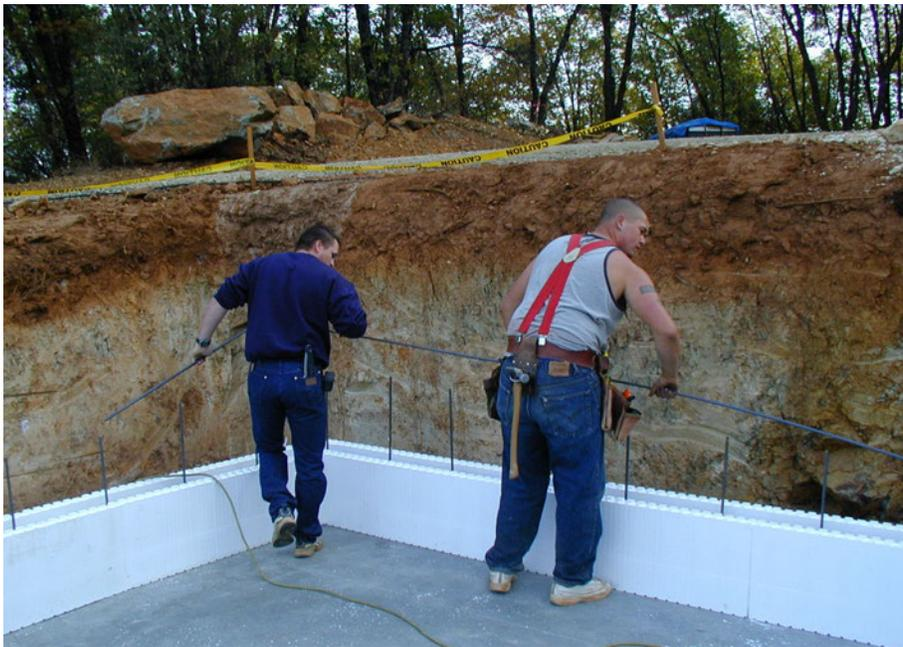
Figure 13 – Installing horizontal rebar
