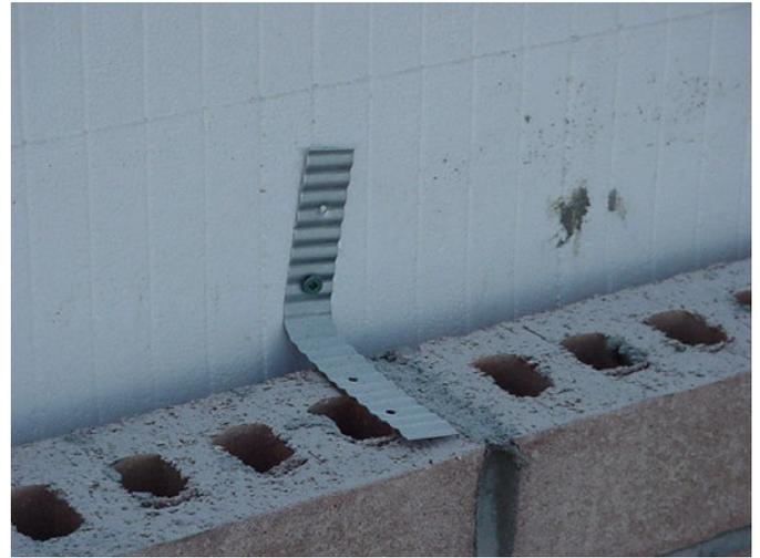
Figure 25 – Standard brick ties screwed into the ICF webs
