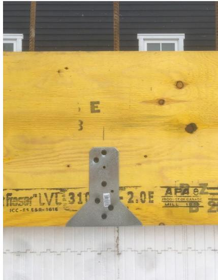
Figure 52 – Laminated Veneer Lumber ledger attached using ICFVL-CW
