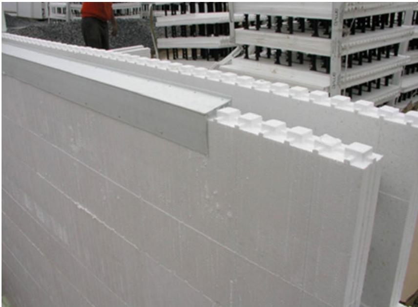
Figure 26 – Protecting the interlock on a top course
