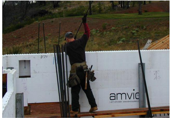
Figure 27 – Installing vertical rebar
