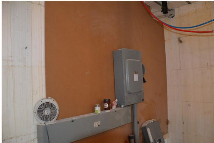
Figure 1 - Electrical panel installed on Amvic™ ICF
