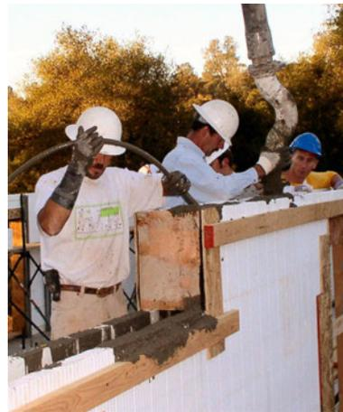
*Figure 10 – Using internal vibrator to consolidate concrete*
