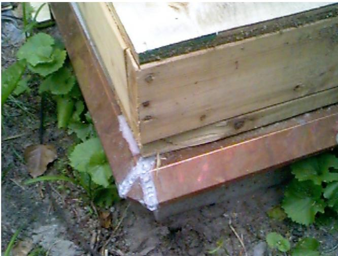
Figure 9 – Metal termite shield using copper metal on top of foundation wall
