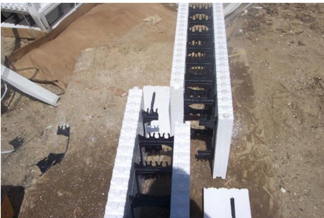
Figure 5 – Setting the two cut forms into position
