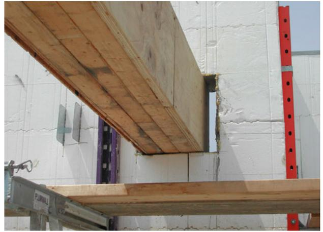
Figure 57 – Once the concrete is cured sufficiently, void fill is removed, and beam is installed
