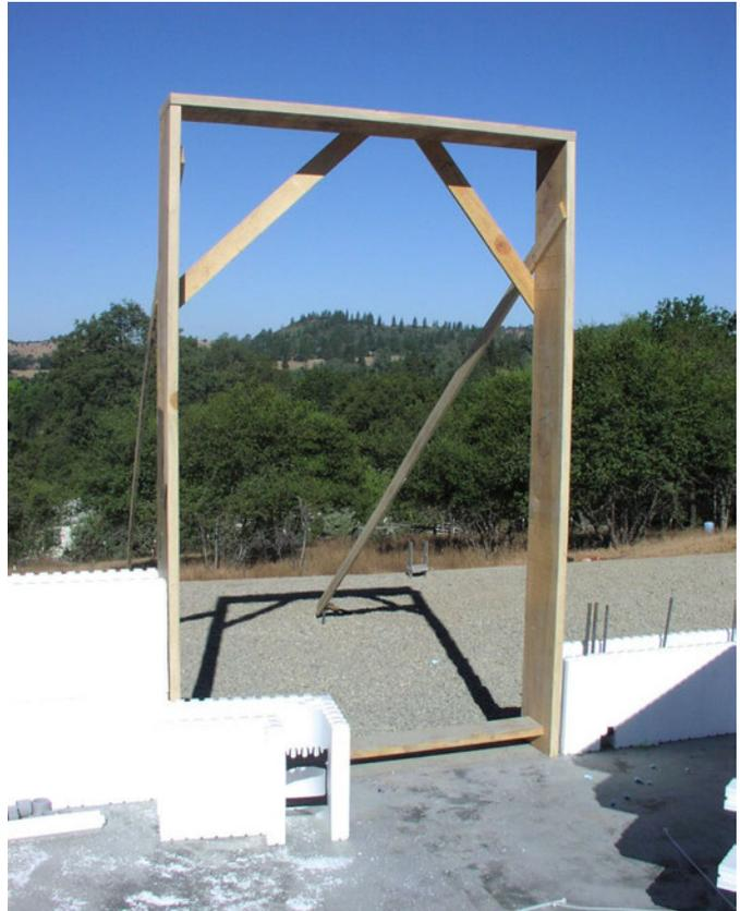
Figure 7 – Placing Door Bucks
