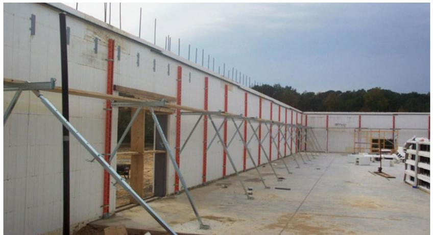
Figure 29 – Bracing on the inside of the wall
