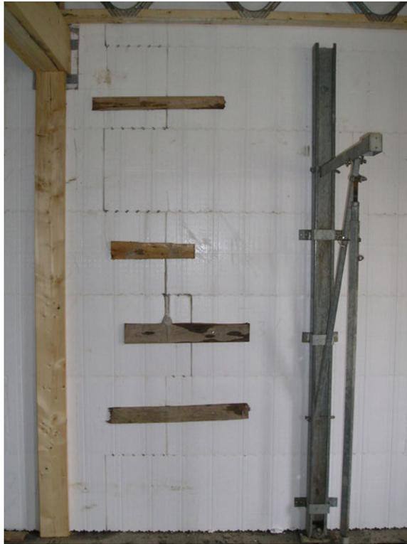
Figure 39 – Additional bracing when vertical joints are less than 6in (152mm) apart
