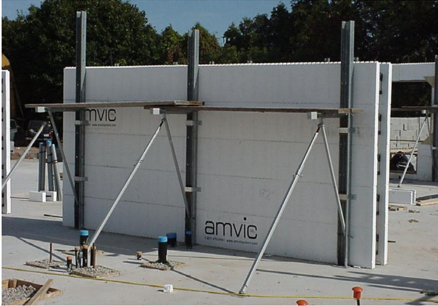
Figure 30 –Platform and scaffold planks
