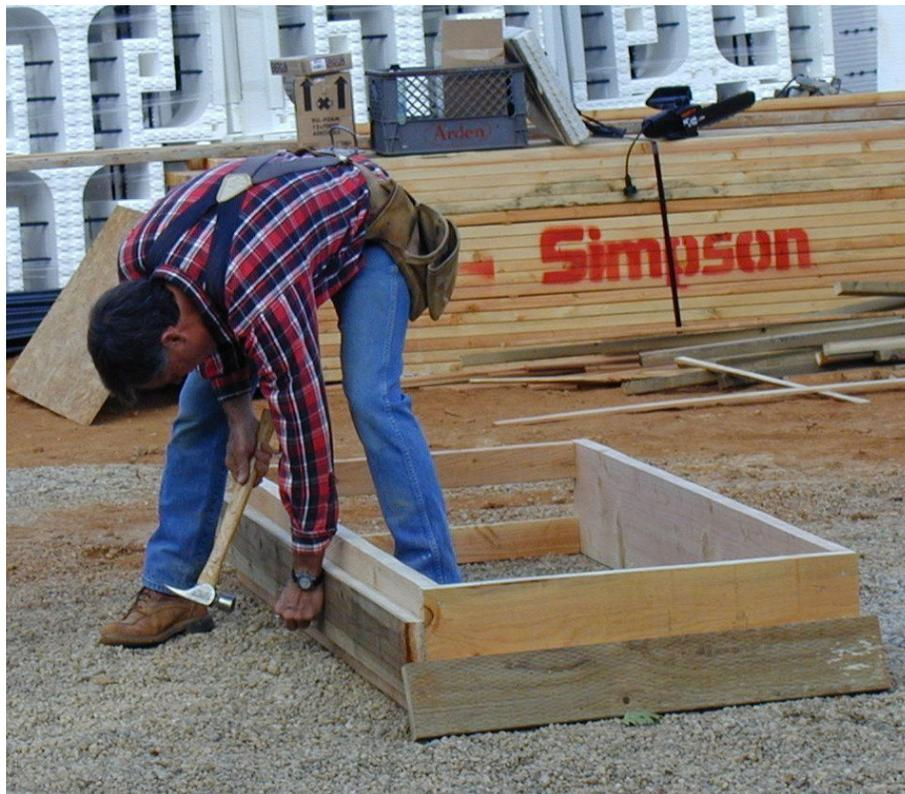
Figure 1 – Constructing your window/door bucks
