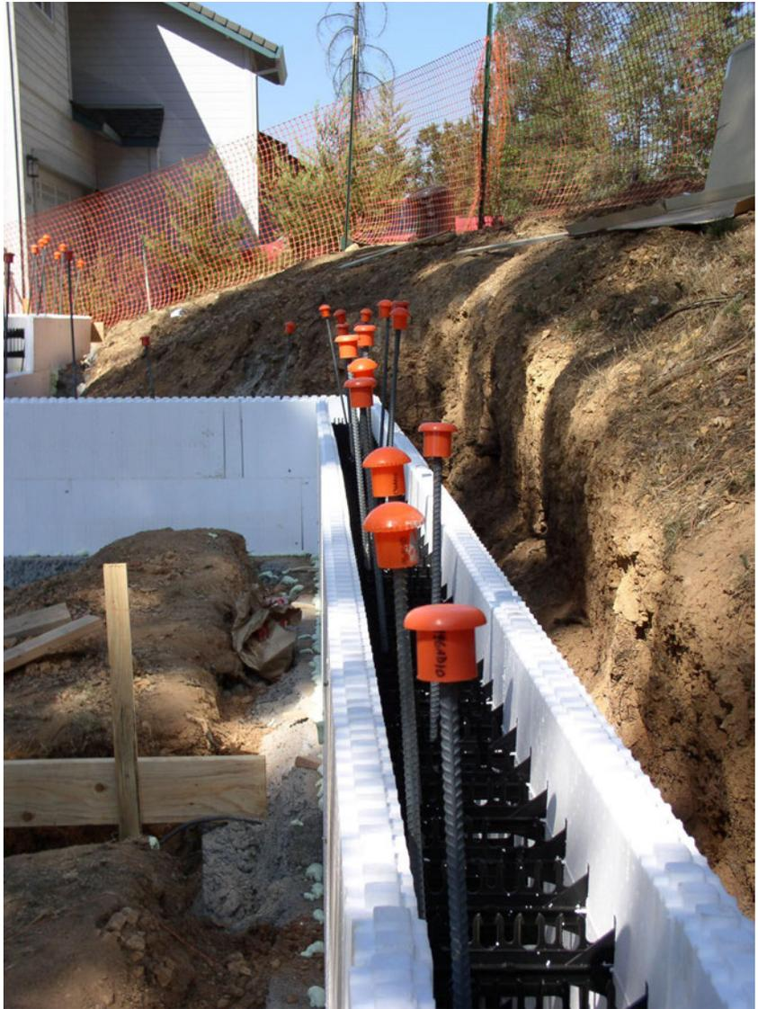
*Figure 5 - Plastic mushroom caps on protruding steel bars*
