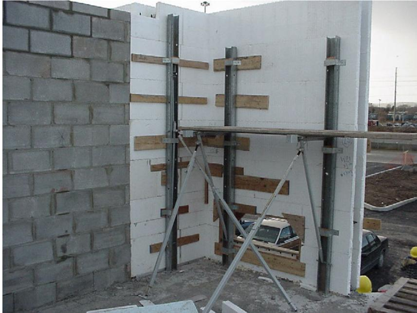
Figure 32 – Bracing corners on the inside
