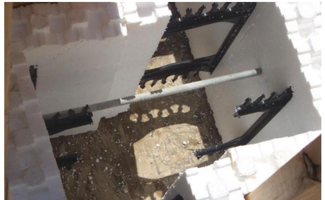
Figure 9 – Threaded rod inserted through both wood forms
