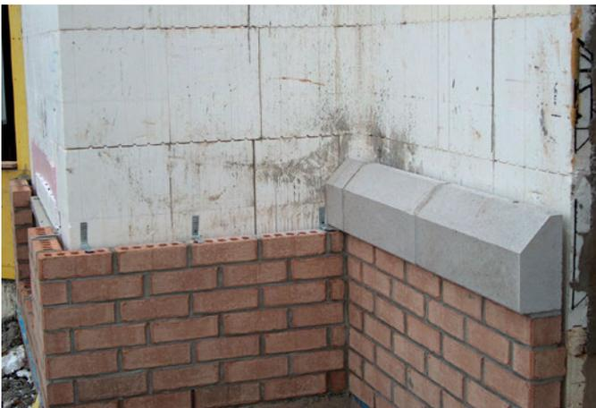
Figure 4 – Brick veneer construction with Amvic™ ICF
