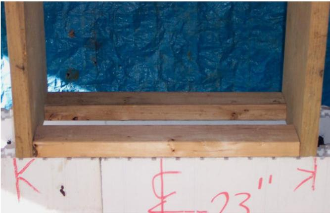
Figure 4 – Typical full width window buck bottom construction
