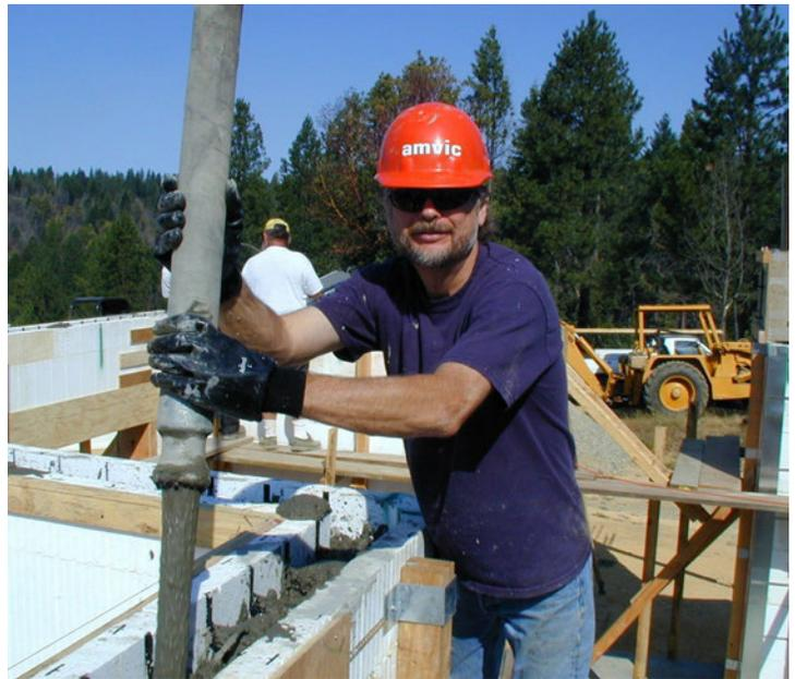
Figure 9 – Pour concrete in lifts of 3-4' (0.9-1.2m)
