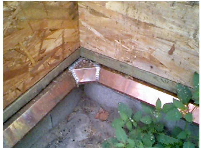
Figure 10 – Detail of metal shield at inside corner
