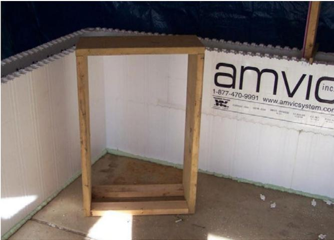
Figure 2 – Typical full width wood buck made of pressure treated lumber
