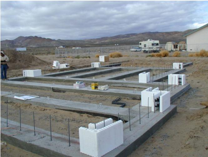
Figure 8 – Placing corner block first
