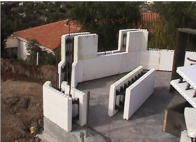
Figure 15 – Reversing 45° corner blocks for bay window
