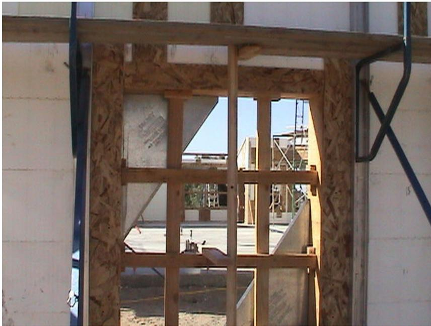
Figure 37 – Bracing wall opening vertically and horizontally
