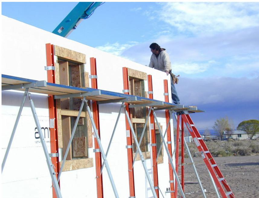
Figure 33 – Bracing both sides of wall openings
