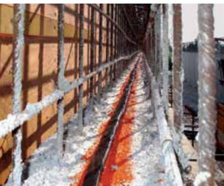
**PENEBAR PRIMER** is applied first to the area where the waterstop is to be placed. It is quickly and conveniently applied at the job site by a simple brush application.
