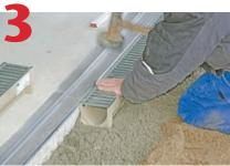
Lay channels starting at outlet. Set a string line at required height to ensure level. Seal joints if required.
