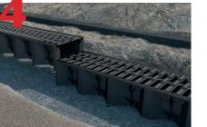
Continue to lay channels working away from outlet, channels slide-fit together.
