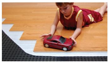
Virtually all basements have moisture problems. That's because moisture is continually released into homes through the concrete beneath the floor covering. Platon creates a moisture proof barrier and air gap between the floor and concrete, protecting the floor covering while allowing the concrete to breathe and the moisture to vent. As a result, the finished floor stays dry and warm, without build-up of mould, mildew or odours that affect the floor covering's lifespan and indoor air quality.
