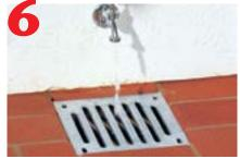
Ensure finished surface is 1/8" higher than the grate to assist water drainage.
