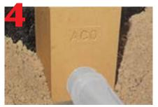
Connect drainage pipe, check for leaks before backfilling.
