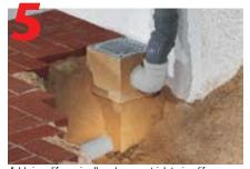
Add riser (if required) and connect inlet pipe (if required). Surround PointDrain with good quality concrete. Finish with surfacing material.
