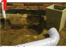
Dig hole to fit PointDrain and necessary pipe-work.
