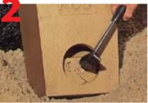
Drill out/cutout holes for pipe connection.
